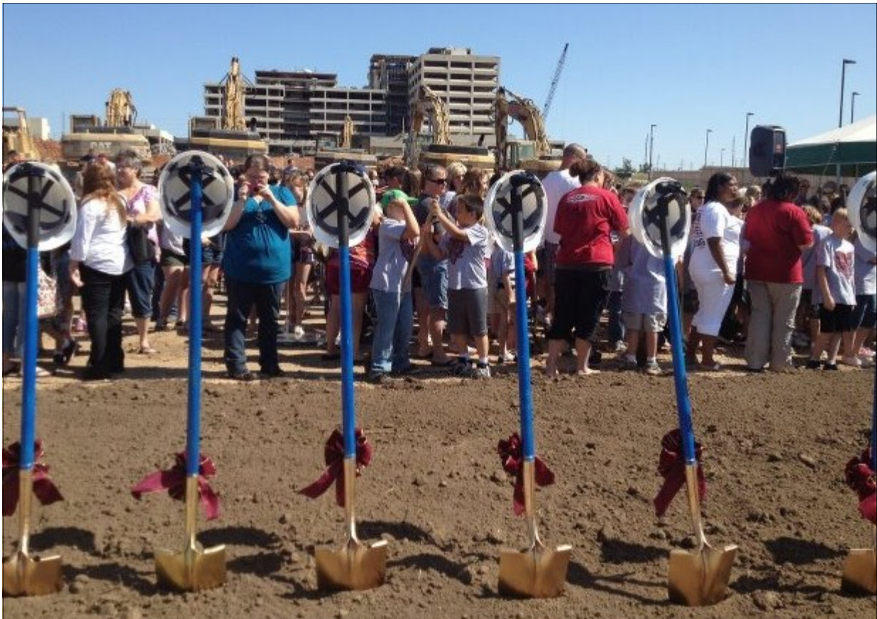
Groundbreaking for Irving Elementary in Joplin on one-year anniversary of the tornado there. Note the former St. Johns Hospital in the background which is in the process of being torn down.
